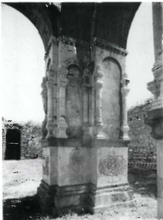
St. Tadeos, Bell tower, Southwestern pillar; photo by A. Haghazarian.
